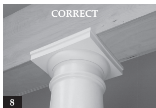
8. Remove any bracing and allow the load to bear on the column shaft. Make sure the load is centered over the entire circumference of the column shaft. When in proper position: (a) The top and bottom of the column shaft will fit evenly with the adjoining surface. There will not be any voids or distortions between the shaft and the adjoining surface. (b) The load will rest evenly around the entire circumference of the column shaft. NOTE: Do not finish the installation unless both (a) and (b) are achieved.
