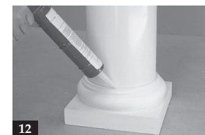
12. Apply a paintable silicone caulking between the base and the shaft. (Note: Not all silicone caulking is paintable.)
