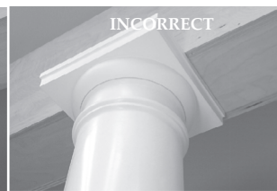
8. Remove any bracing and allow the load to bear on the column shaft. Make sure the load is centered over the entire circumference of the column shaft. When in proper position: (a) The top and bottom of the column shaft will fit evenly with the adjoining surface. There will not be any voids or distortions between the shaft and the adjoining surface. (b) The load will rest evenly around the entire circumference of the column shaft. NOTE: Do not finish the installation unless both (a) and (b) are achieved.
