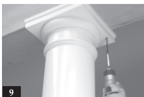
9. Slide the capital into place and pre-drill through the capital and shaft. Install with rust resistant screws. Use automotive body filler to cover the screw heads.
