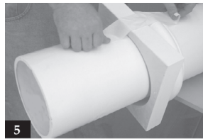
5. Slide the base onto the column shaft from the bottom. It may be necessary to hold the base in position with tape.
