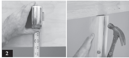
2. Measure the overall opening height. Raise the soffit slightly with a sturdy brace to allow positioning of the column during installation.
